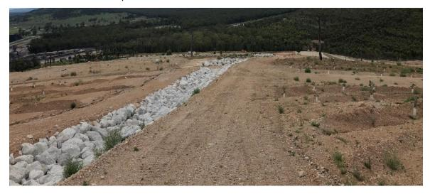
Figure 17 - Photo: Rocklined Drop structures on the Northern Rehabilitation area
